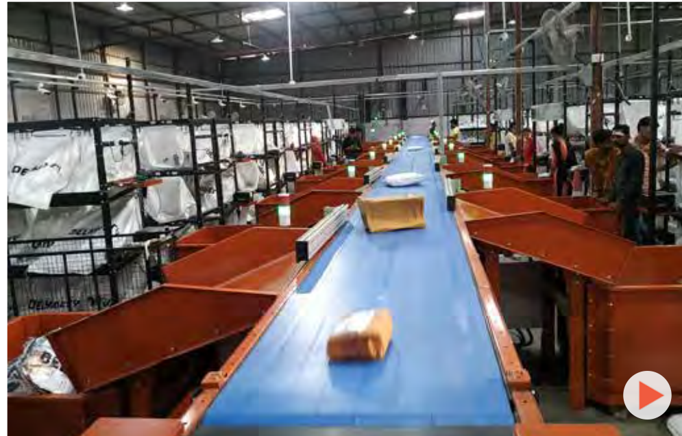
Linear arm sorter with put to light system Primary and secondary sorting | Industry: 3PL
